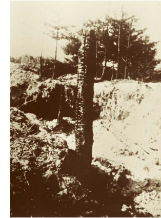
The remains of the burnt-down forest hut at Kyjanice (The Ethnological museum in Olomouc)
